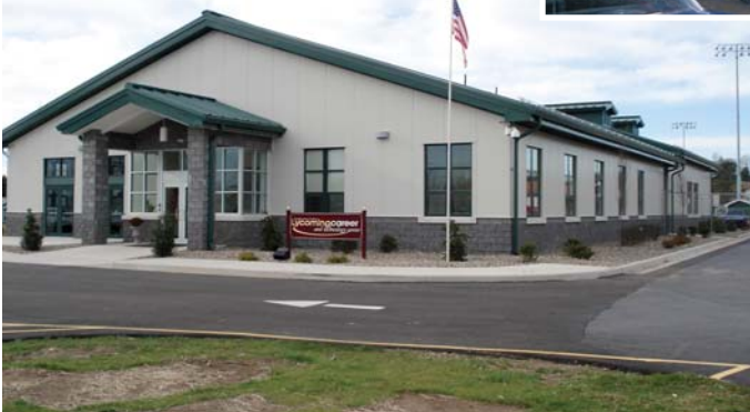
Project: East Lycoming Career Center Location: Hughesville, Pennsylvania Builder: BK Structural Systems
