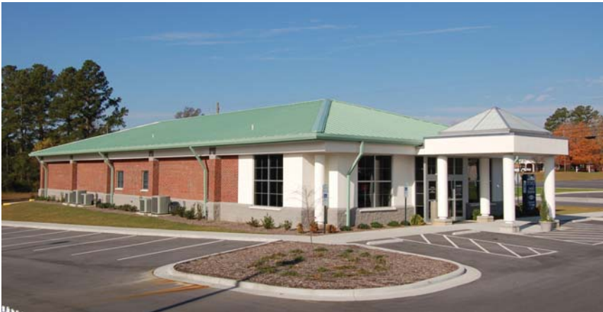
Project: Clinton Medical Clinic Annex Location: Clinton, North Carolina Builder: H. N. Carr, Inc.
