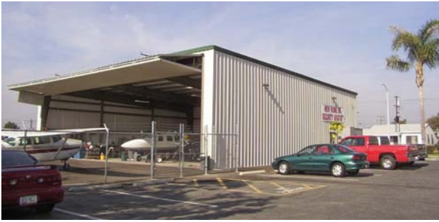
Security Aviation Hawthorne, California G & W Builders, Inc., Builder
