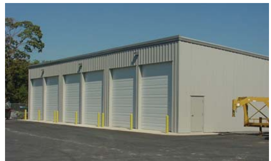
TPWA Light Plant Tahlequah, Oklahoma Girdner Construction, Builder
