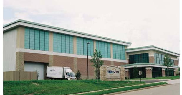
MTM Corporate Headquarters Verona, Wisconsin TJK Design Build, Inc., Builder
