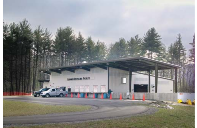
Lebanon Transfer Station Lebanon, New Hampshire Construx, Inc., Builder
