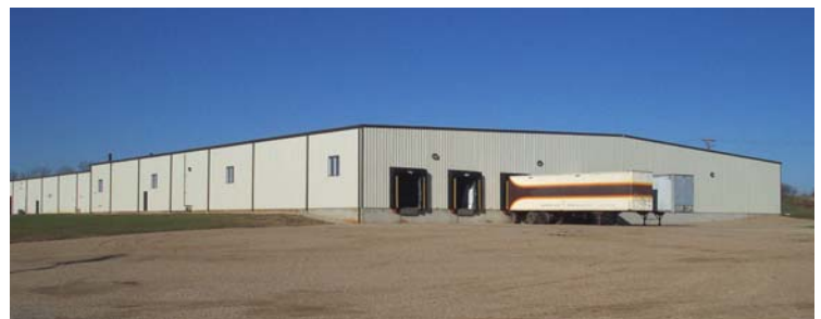
Versa-Tech Fredericktown, Missouri Sargent Construction Company, Builder
