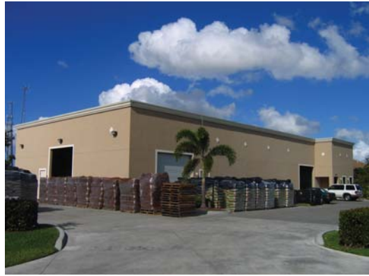
American Fertilizer Naples, Florida Tamiami Builders, Inc., Builder
