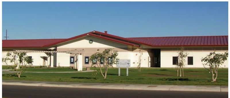
Seabee Training Facility Port Hueneme Naval Facility, California G & W Builders, Inc., Builder
