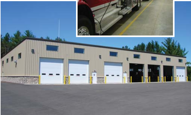
Stockton Garage/Fire Station Custer, Wisconsin Wanta & Son, Inc., Builder
