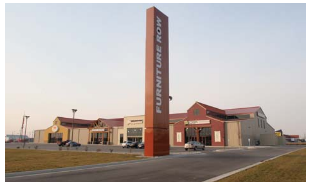
Furniture Row Grand Chute, Wisconsin Furniture Row USA, LLC, Builder
