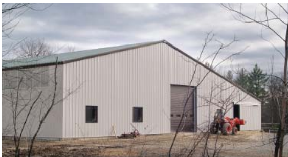
Londonderry Riding Arena Londonderry, New Hampshire Construx, Inc., Builder
