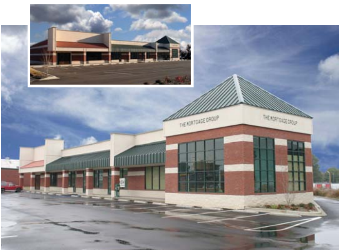
Northside Commons Albertville, Alabama Don Spurlin Construction, Inc., Builder
