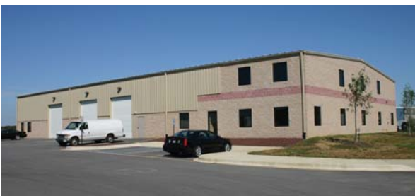
Parkway Floors Middletown, Delaware Nowland Associates, Inc., Builder
