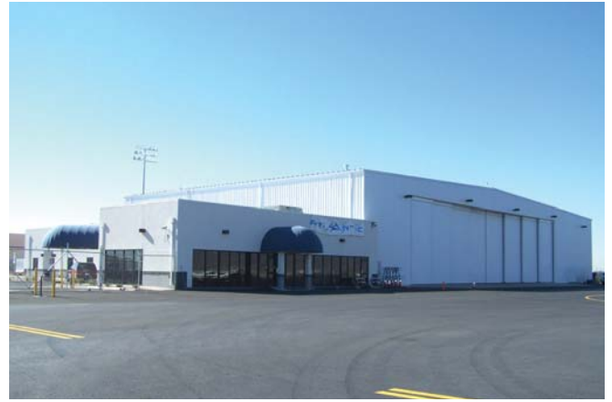
Project: Atlantic Aviation Location: El Paso, Texas Builder: Blair-Hall Company, Inc.
