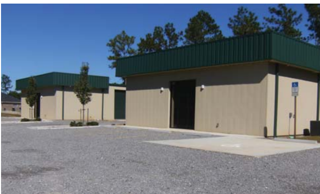
Ward Basin East Milton, Florida Cassida Construction Co., LLC, Builder
