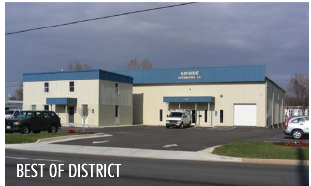
Project: Airside Distributing Company Location: Danville, Virginia Builder: Hughes & Atkins Construction Co., Inc.
