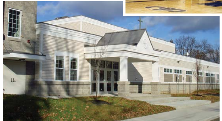
Schenectady Christian School Gym Scotia, New York United Progress, Inc., Builder
