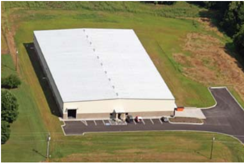
Electro-Mavin Riceville, Tennessee Wilson Construction Group, Builder
