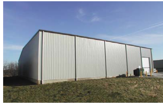
DeJong Manufacturing North Addition Sharon, Iowa Bushong Construction Company, Inc., Builder
