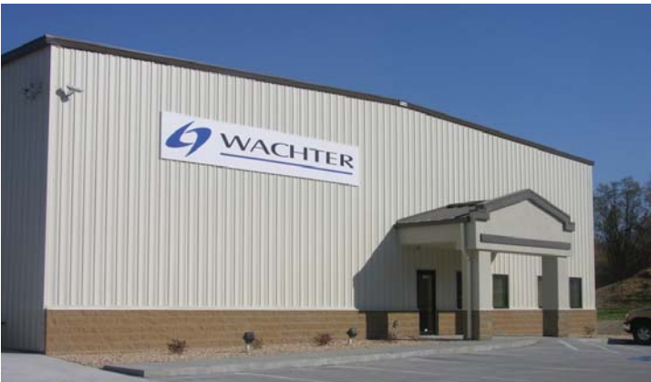
Wachter Electric St. Joseph, Missouri Al J. Mueller Construction Company, Builder
