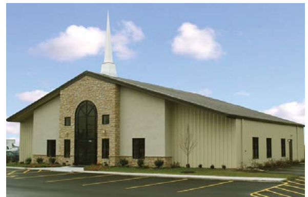
Templo Cristiano Emanuel Church Columbus, Ohio Maverick Builders, Inc., Builder
