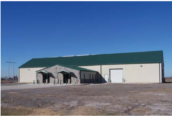
Owens Project Royse City, Texas Rafter P Construction, Inc., Builder
