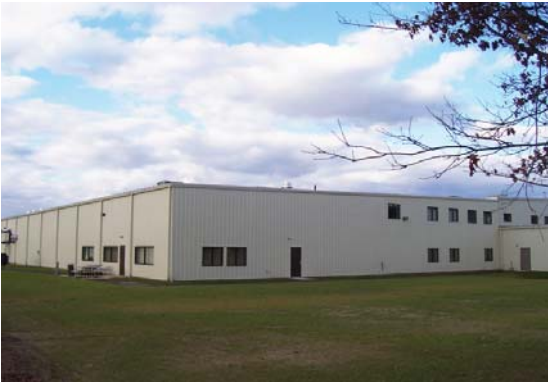
Governors America Corporation Agawam, Massachusetts Forish Construction Co., Inc., Builder
