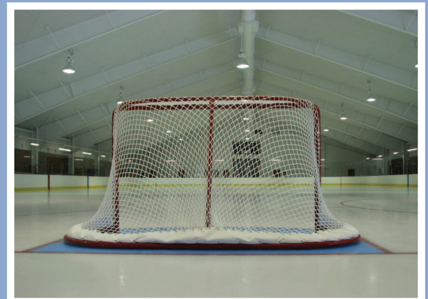
Lufkin Ice Rink Washington Depot, Connecticut Fortunato Construction Group, Inc., Builder
