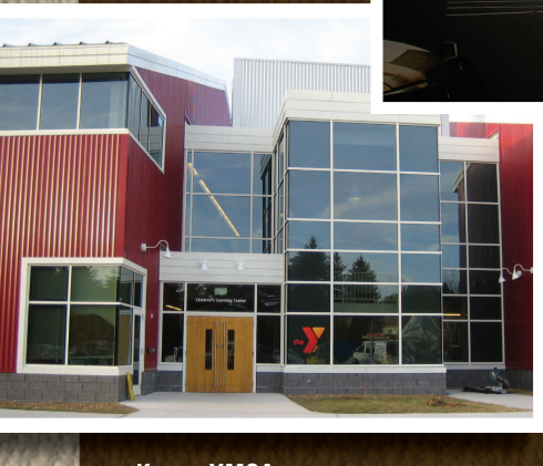
Keene YMCA Keene, New Hampshire Landmark Erectors, LLC, Builder
